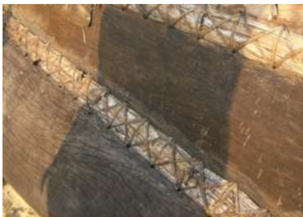
Fig. 8 Stitching with the ‘envelope-flap design’
