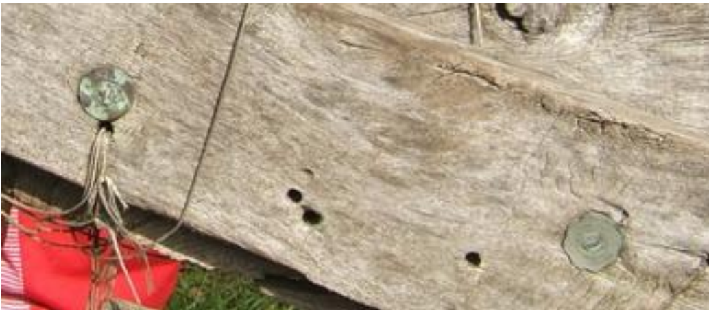
Fig.12 Use of coins and nails for quick repair
